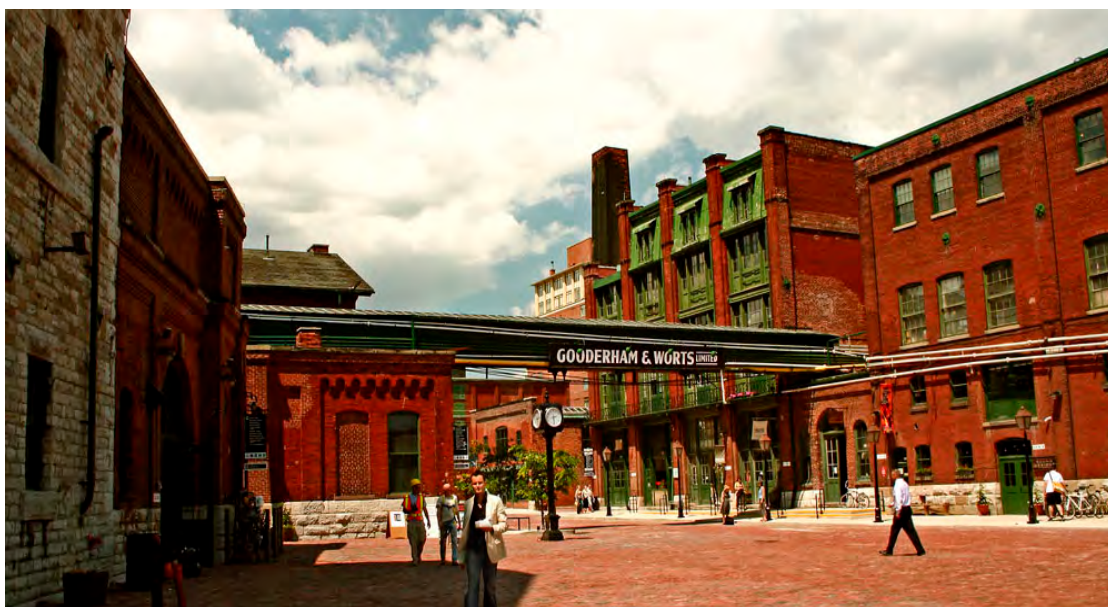
Historic buildings can be converted to other uses to create vibrant urban space.
